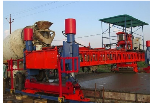
HYDRAULIC DRIVEN BOGIE
